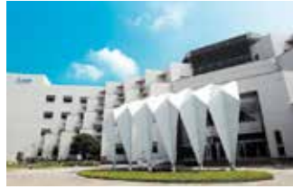
Tainan Plant (Diamond-rated Green Building)
