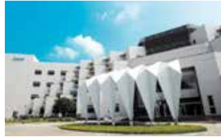
Tainan Plant (Diamond-rated Green Building)
